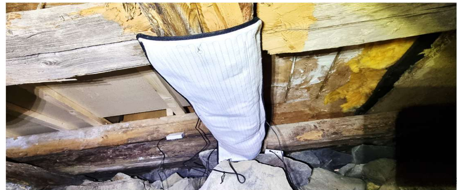
InfraVivo IR Drying Blanket - field test in a Log wall
