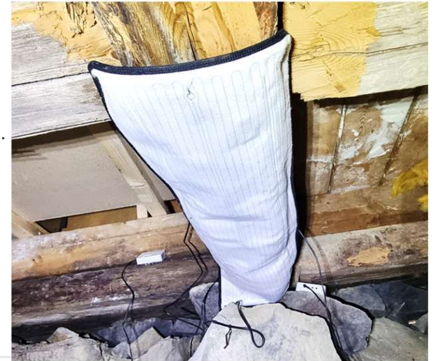
InfraVivo IR Drying Blanket - field test in a Log wall
